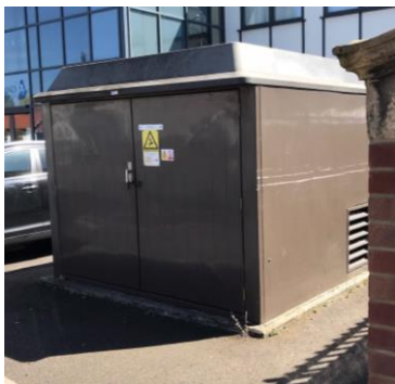
Typical GRP Substation
