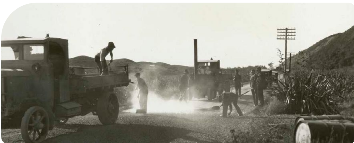
Creator unknown: Photograph of workers sealing the Paekakariki-Paraparaumu road.
