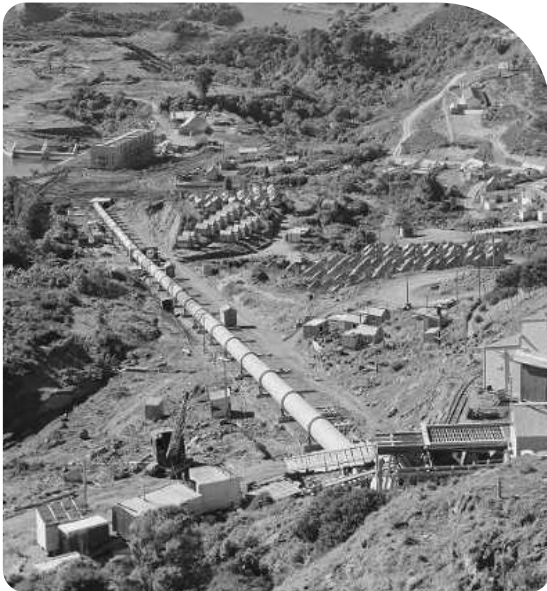
Kaitawa hydro electric power station under construction, at Waikaremoana. Tourist and Publicity.
