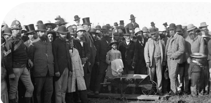
Digging the first sod for the Main Trunk Railway, at the confiscation line at the southern bank of the Puniu River. Beere, Daniel Manders, 1833-1909: Negatives of New Zealand and Australia.
