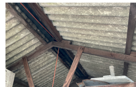
Asbestos cement roofing sheets on garage
