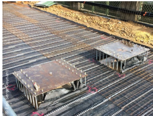
Luxembourg line 1, installation of a track with spring vibration isolators
