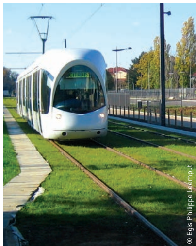
Lyon T3 - Rhônexpress, embedded grass-covered ballast track, mixed urban and railway section
