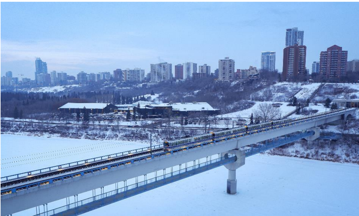
A light rail line designed for temperatures that can drop to -40^{\circ}\text{C} for several weeks
