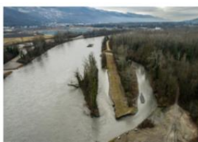
Setback of the embankment, opening up of the existing structure and reconnection of a backwater (Lumbin) ©SYMBHI
