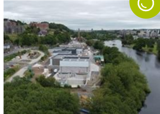
Lee Road Water Treatment Plant Upgrade Cork – Ireland
