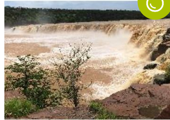
Gouina Hydroelectric Generating Station Mali
