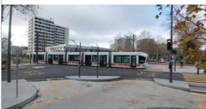
Safe traffic control at a Dutch-style junction: LRVs and bikes pass alternately
