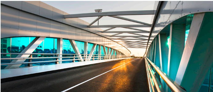
Yas Marina Hotel Access Bridge UNITED ARAB EMIRATES
