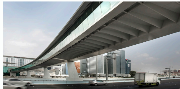
Abu Dhabi National Exhibition Centre Bridge UNITED ARAB EMIRATES
