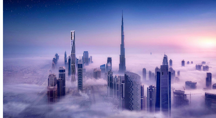
SRG Residential Tower
