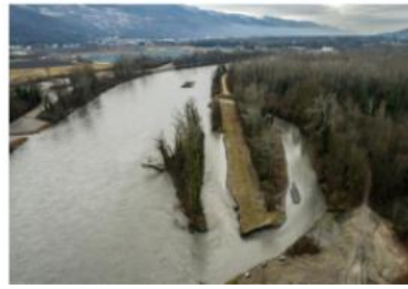
Levee setback, opening of existing levees, and reconnection of an abandoned river channel (Lumbin)©SYMBHI
