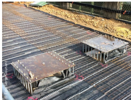
Luxembourg line 1, installation of a track with spring vibration isolators
