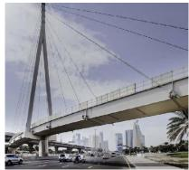
The design and built of the cable-stay bridge which consists of a long main support suspended from a tower with inclined hangers. The towers can be designed in numerous ways and the cables can be fixed in a fanshaped or harp-shaped arrangements. As with suspension bridges, guarding against wind-based vibration is extremely important.
