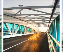
Design and built of the only land connection to the Marina Hotel, which is surrounded by the Formula 1 racetrack. This special bridge consists of two reinforced earth walls, a steel Warren Truss Bridge and a streamlined composite panel cladding with lighting and two
