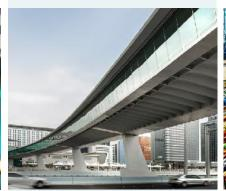
Fabrication of the ADNEC Bridge from 600 tons of steel and 132 glazed panels. It is 162 m long and spans all eight lanes of the Khaleej Al Arabi Coast Road adjacent to ADNEC.
